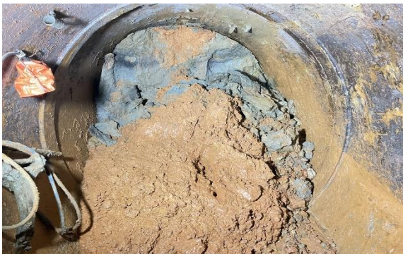
(a) Tunnel face of left gallery pipe
