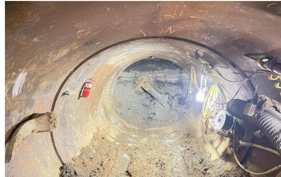
(b) Tunnel face of right gallery pipe
